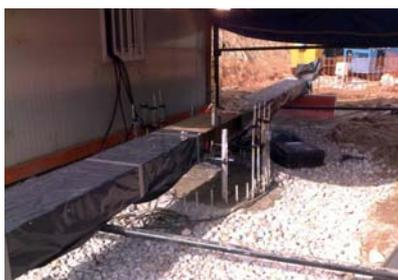
O-cell bi-directional testing setup
